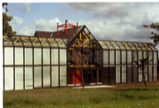
The south elevation makes the most of winter gains by heating the roof so that in the cold fully glazed the cavity is double height and provides an option for naturally and heated air to be transferred to the production area in winter or summer.
