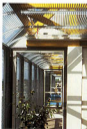
The glazed walls and rooflights use thin, soft internal blinds. It was thought that Poly flux tubes fit between the blinds giving even an even flow of the light. The blinds are motorised and the false ceiling was omitted on the walls to prevent a hot floor when the heat is turned on during business hours.
