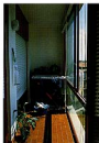
Roller blinds are fixed to the glass doors onto the sunspace, and reflective venetian blinds are mounted behind the external glazing. Both devices assist to reduce glare.
