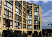
Fully glazed south facade creates balconies for each flat across the full width. All the windows have pre-cast red steel frames and are draughtstripped.
