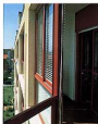
Interior view of the glazed balcony in a corner apartment. The upper part of the glass covers off existing windows while the lower part forms the balcony (parquet).
